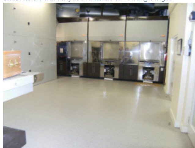
View of the crematory with the Evans 300/2 cremators installed in 1997 and on the left the screen around the retrofitted filtration plant installed in 2011. The screen is for aesthetic reasons when mourners come into the crematory to witness the coffin being charged.
