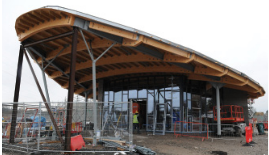
Canopy and glazed entrance to the waiting area and chapel under construction
