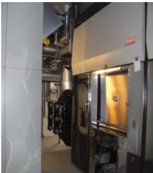
Cremator No.2 and to the immediate left of it can be seen the end of the boiler which was slotted into the space vacated by the redundant No.1 cremator. To the very left is the edge of the screen surrounding the filter which stands in the space previously required to charge No.1 cremator.
